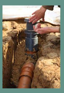
A plan for the overflow system must be established. In this case the water storage area was connected to an existing soak away. An alternative option is to transfer the water to another storage area, such as an intermediate water storage tank.
