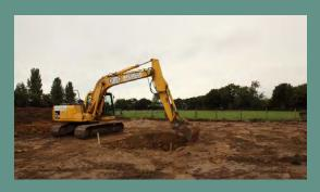
After the top soil is removed, the initial rectangular dig area can be marked out using poles and liner-marker, then excavation can begin. Once the initial rectangular section is complete, slopes can be built out from this area.
