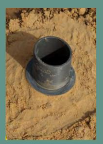
When creating the connection between the overflow and the liner it is essential to align the base of the overflow connection flush with the slope face. This can be done by building up a sand structure around the overflow pipe.
