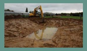
The slopes and sides must be levelled and compacted to create a smooth surface for the liner. For slopes of 1 in 3 rolling machines can be used to compact surfaces to 98% compaction.
