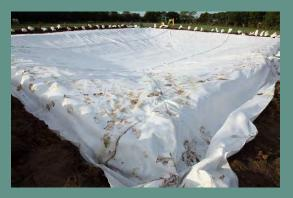
The sandbags can then be put into the anchor trench to keep the underlay in place, until the liner is ready for installation.
