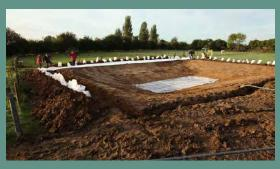
The underlay must be rolled out as per the fabricators stated directions and information on this will be provided by your supplier. It is important to follow these directions as this will allow the simplest method of unfurling. If guidance is not provided contact your supplier before unfurling.
