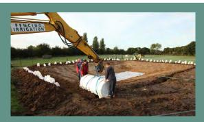
With the site clean, anchor trench dug and sandbags in place, the underlay can be delivered to the site. It is recommended that the underlay be installed in good weather conditions.
