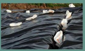
do this evenly across the material and if a strong prevailing wind is expected from a specific direction, additional sandbags may need to be placed in this area.
