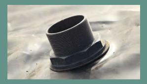
As seen in the demonstrational video, the underlay and liner can be pulled over the overflow pipe and cut accordingly. Care must be taken during this process as a tight seal is required. After this, the liner can be temporally
