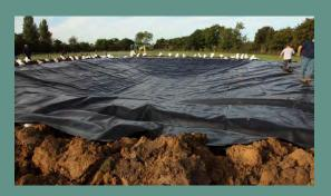
The best method to install the liner is to evenly spread the people across the area and to lift the cover up and down to waft air underneath as this reduces the friction between the cover and the ground. This also allows the liner to be unfurled in several stages. When the liner has been put into place, it can be tensioned by walking the material into the anchor trench.
